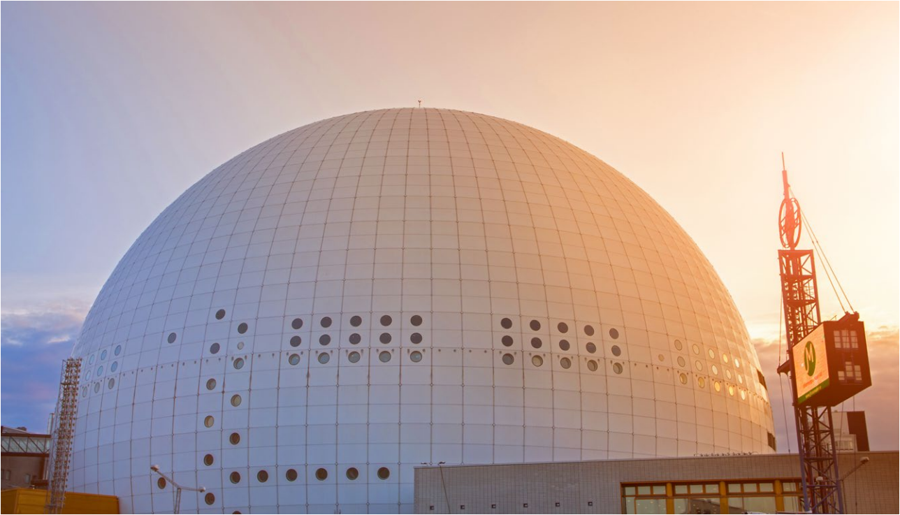
Figure 3 In the Globen Shopping mall 29 lifts use CANopen Lift controllers (Source: Hisselektronik)
