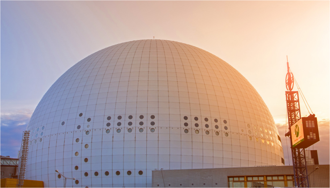
Figure 3 In the Globen Shopping mall 29 lifts use CANopen Lift controllers (Source: Hisselektronik)
